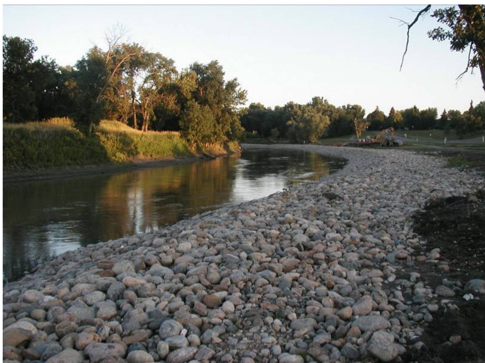
Rocks used to stabilize an outside bend.
