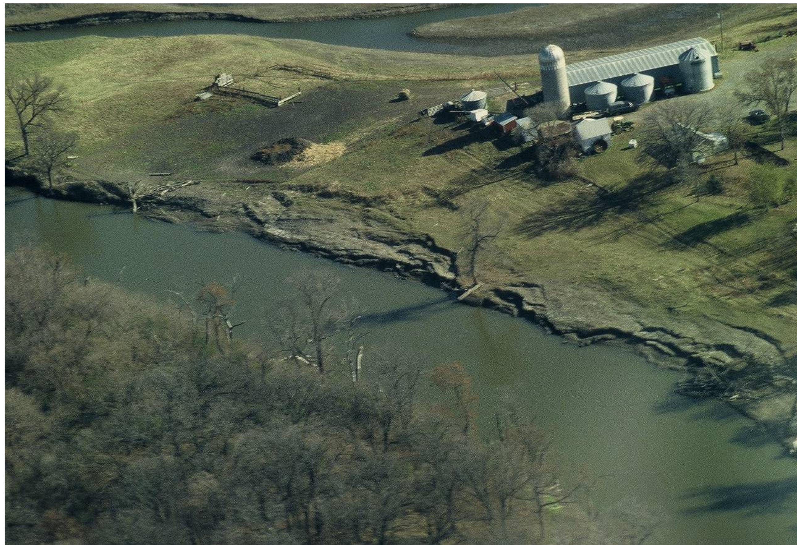
Removal of vegetation often results in riverbank erosion and slumping.
